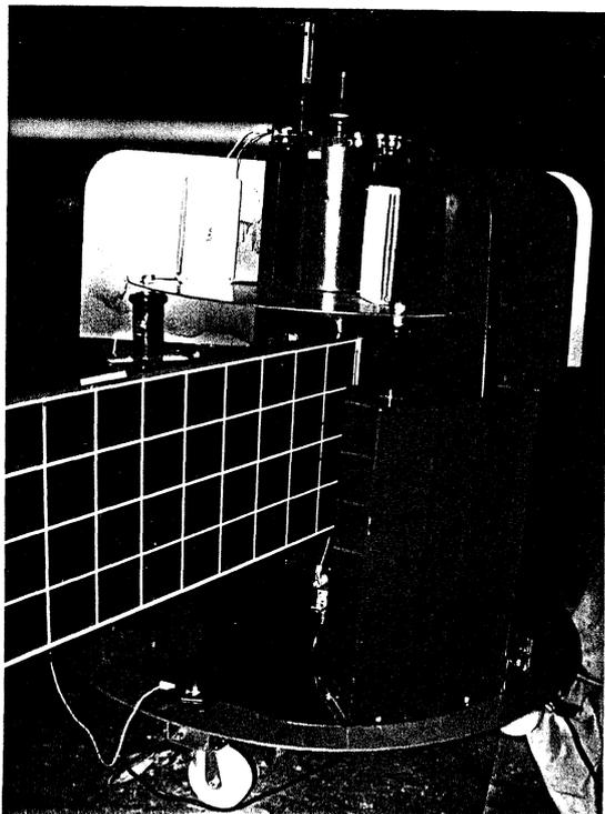
Fig. 2 : Photograph of ISB's high impulse-current generator.
