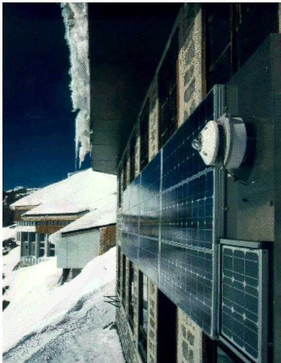
**Fig. 1:** View of the grid connected PV plant (1.1kWp) at the research station at Jungfrauoch (3454m, about 46.5°N): One of the two arrays with irradiance sensor (pyranometer and reference cell).
