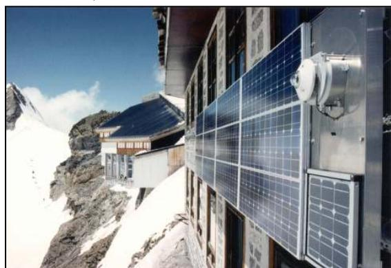
**Fig. 1:** View of the grid connected PV plant (1.1kWp) at the research station at Jungfrauoch (3454m, about 46.5°N): One of the two arrays with irradiance sensor (pyranometer and reference cell).
