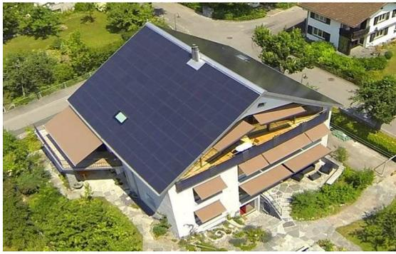
**Figure 6:** Multi-family retrofit house in Switzerland: the roof is an east-west-oriented PV-installation producing 34,6 kWp and a vacuum solar collector for hot water. It covers 187% of the consumption of the house – much more than needed for electric cars or the “grey energy” of the house.
