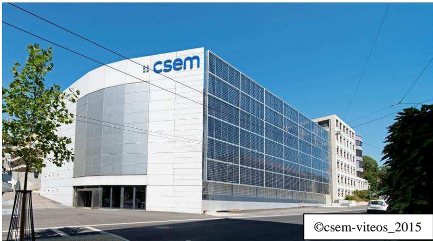
Fig 5: PV-Façade CSEM in Neuchâtel (CH), aesthetical and functional applications promote PV in façades.
