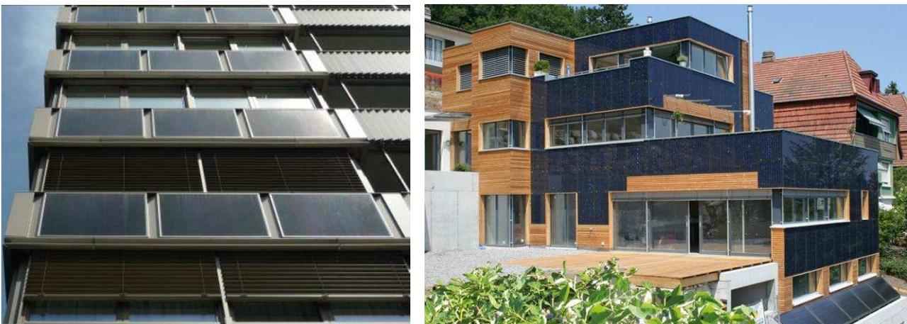
Fig. 7 + 8: Photovoltaic integration with standard sized panels or custom-made panels.
