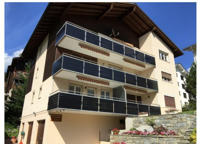
Figure 5: Balcony balustrades can be used to install PV panels vertically and to cut production peaks
